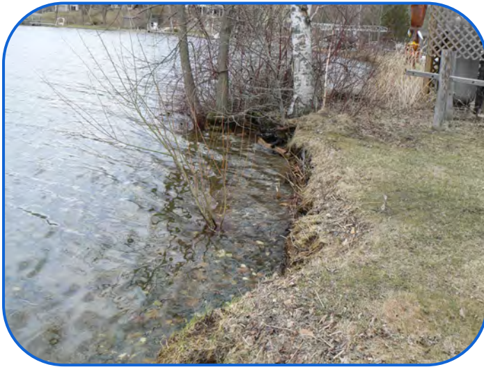
Before Construction of Shoreline
