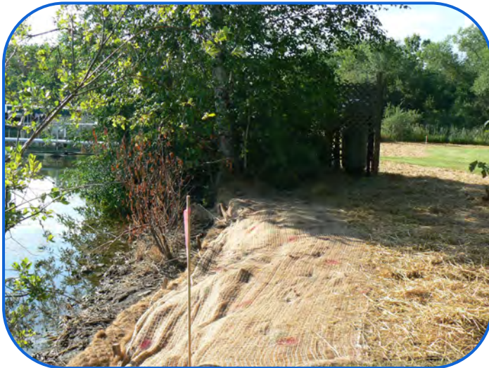
After Construction of Shoreline
