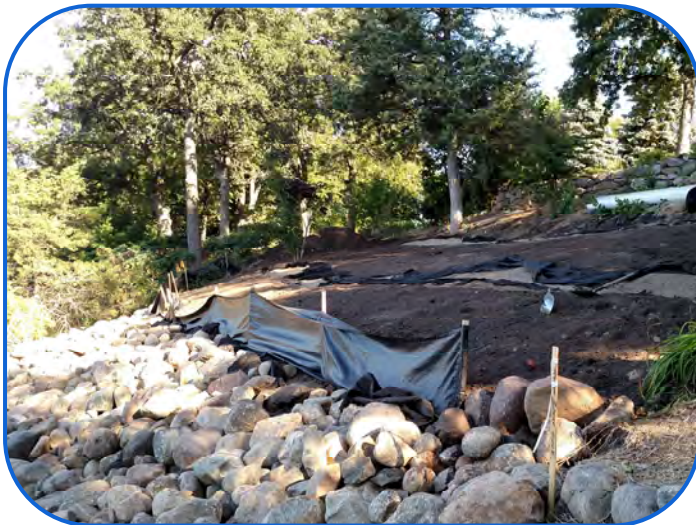
Regraded Slope with Tile Trenches
