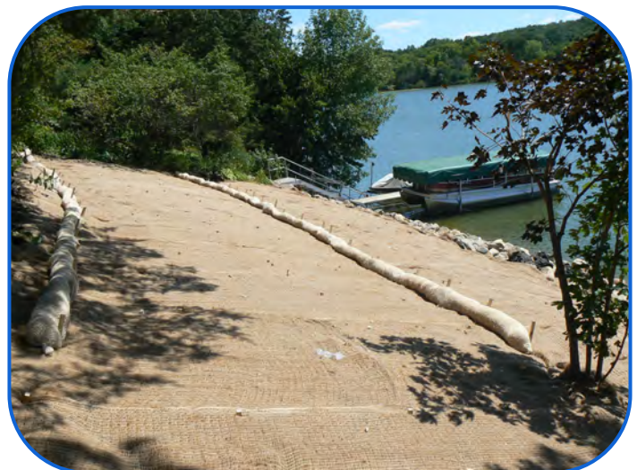
Regraded Slope Prior to Planting
