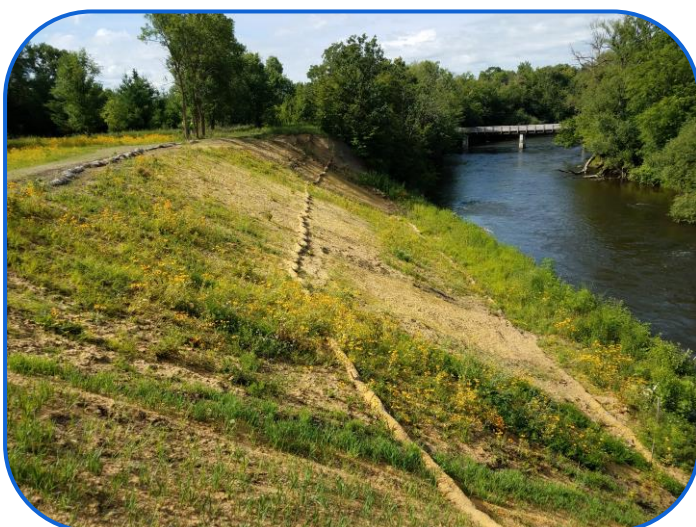
After Streambank Stabilization
