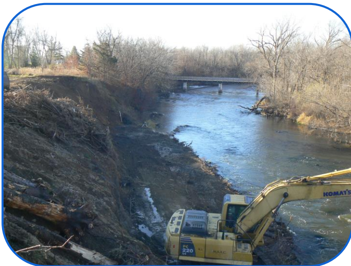
During Streambank Stabilization
