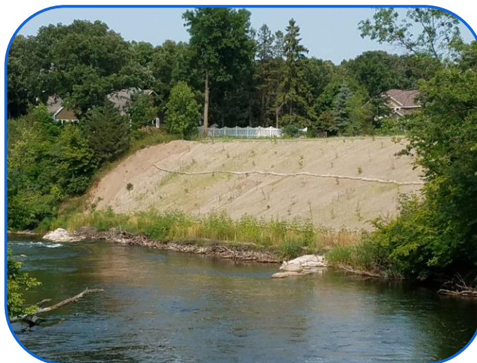
After Streambank Stabilization
