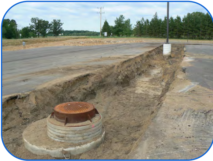
During Construction of a Raingarden
