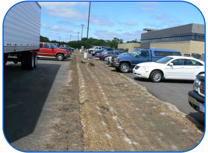
Raingarden with Erosion Control Blanket
