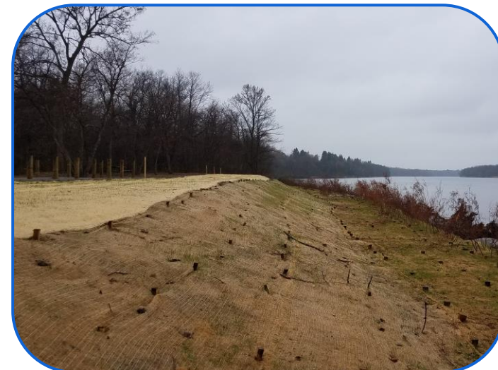
Project Site Prior To Final Planting
