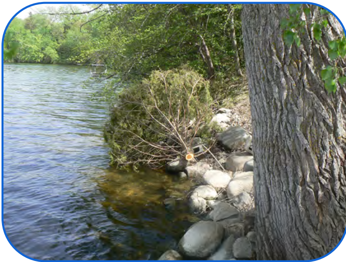
Cedar Tree Revetment Installation
