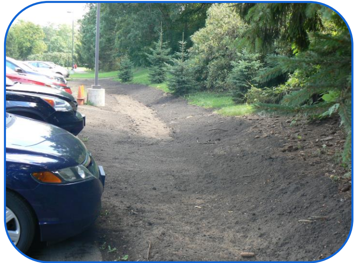
Infiltration Trench Along a Parking Lot
