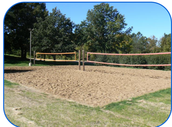
Volleyball Court Amended to an Infiltration Basin
