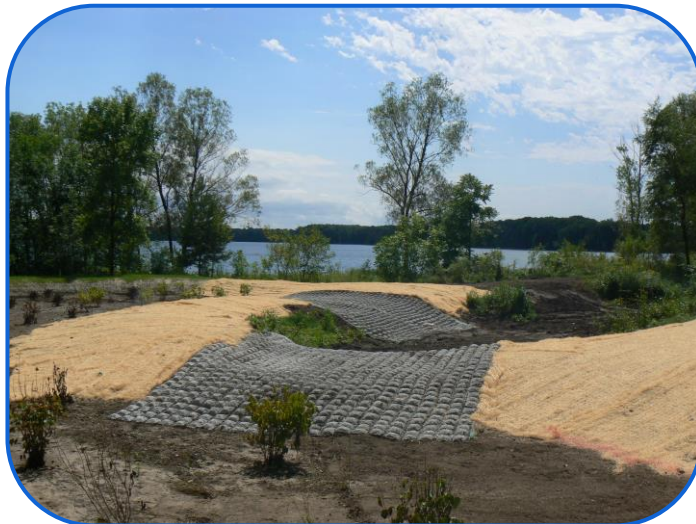
Water Diversions/Infiltration Basins (Before)
