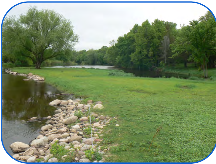
Failing Retaining Wall System
