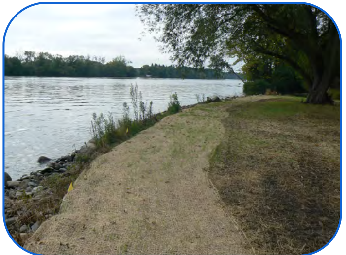
Erosion Blanket & Planting
