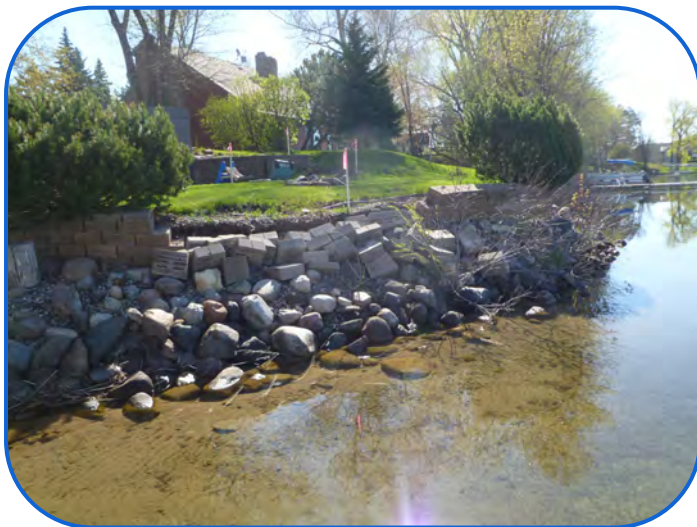
Before Shoreline Restoration & Wall Removal
