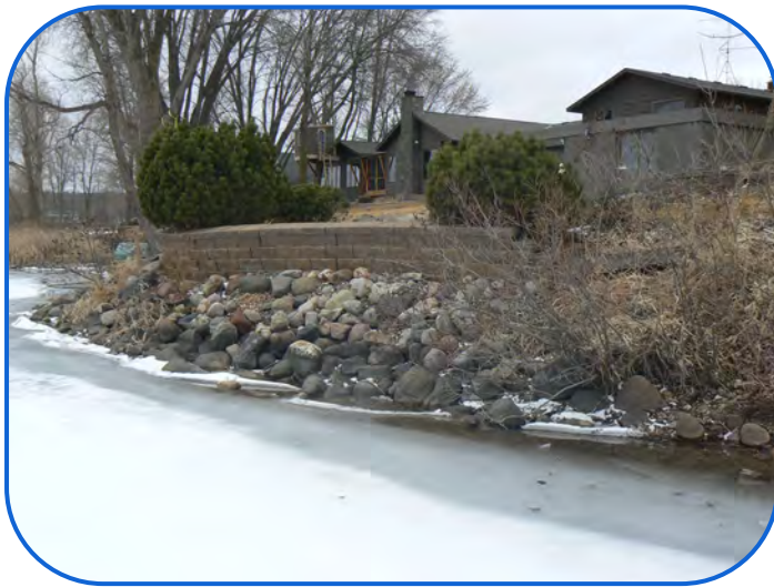
Before Shoreline Restoration & Wall Removal
