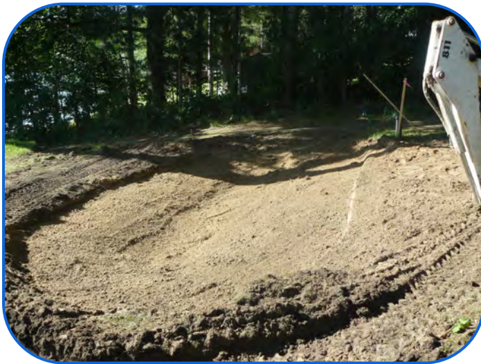
Raingarden During Construction
