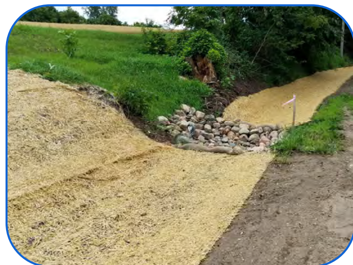
Waterway & Outlet Along Road
