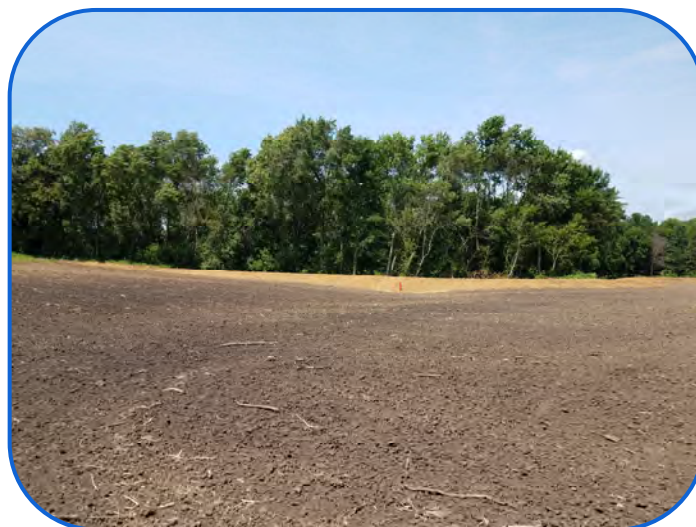
Constructed Basin In Field
