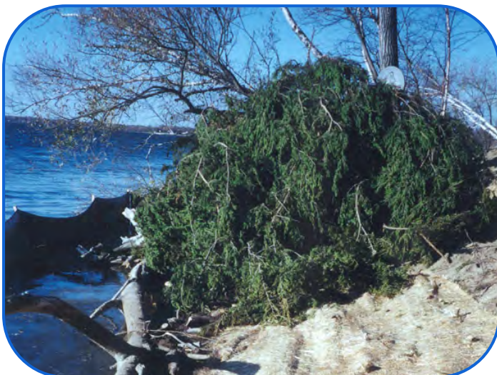
Revetments, Blanket and Stakes
