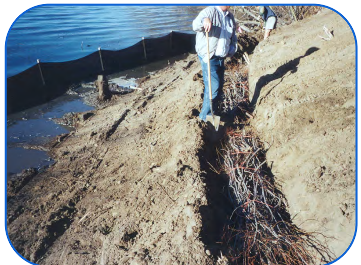
Willow/Dogwood Brush Bundle Installation
