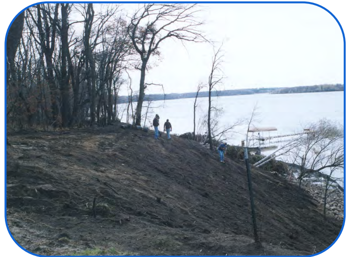
Project During Construction
