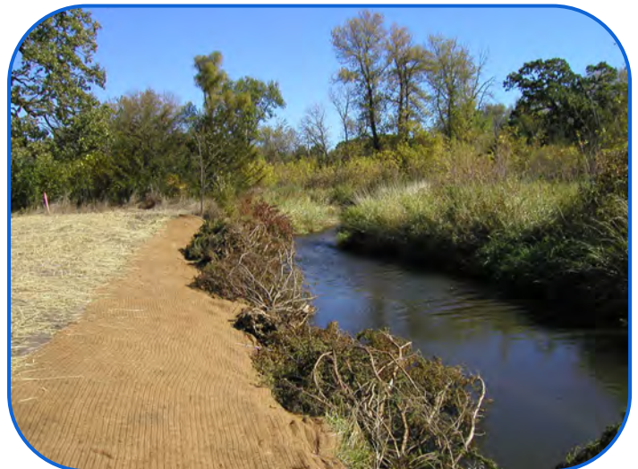
Project After Completion
