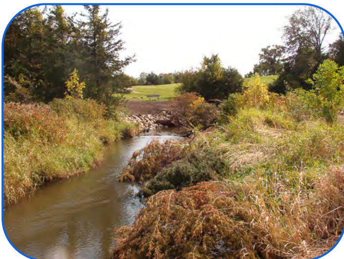
Project After Completion
