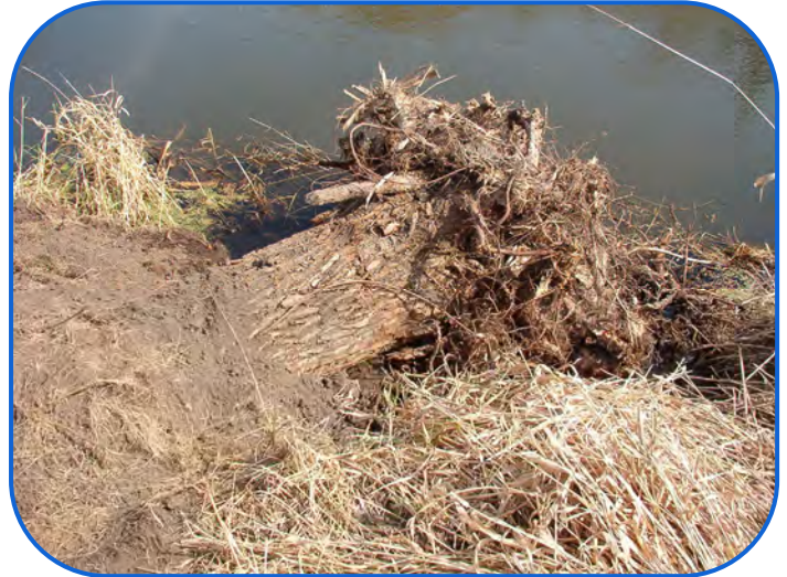
Root Wad Installation
