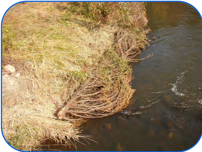
Cedar Tree Revetment Installation
